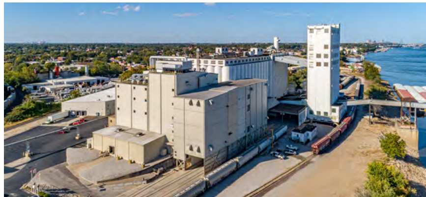
Durum Milling Facility 📍 ST. LOUIS, MO, US
